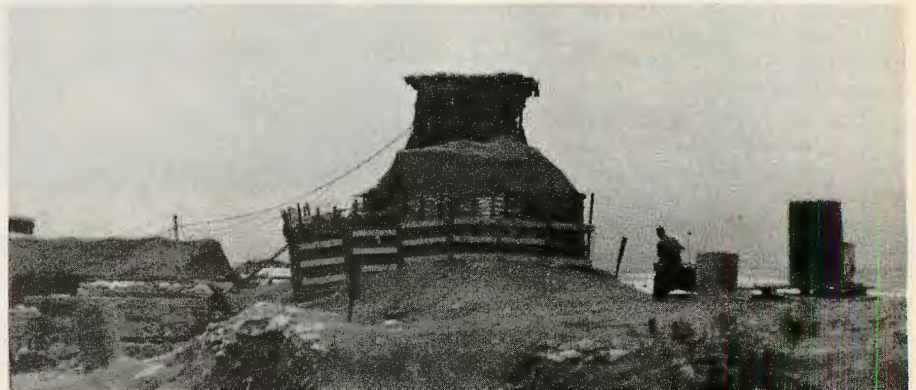
Bunker and tower in which IOD Spyglass Alpha was located on Hill 65.
